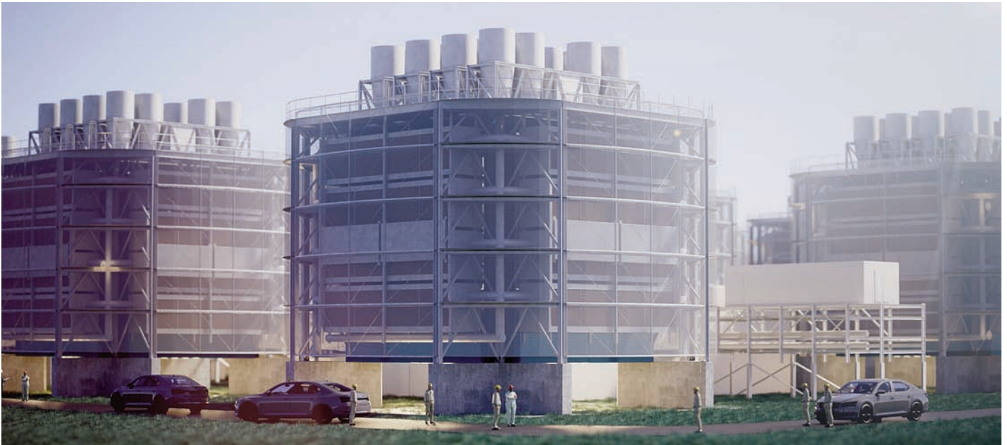
The Generation 3 direct air capture technology is based on novel structured sorbent materials housed in modular cubes (Image: ©Climeworks)
