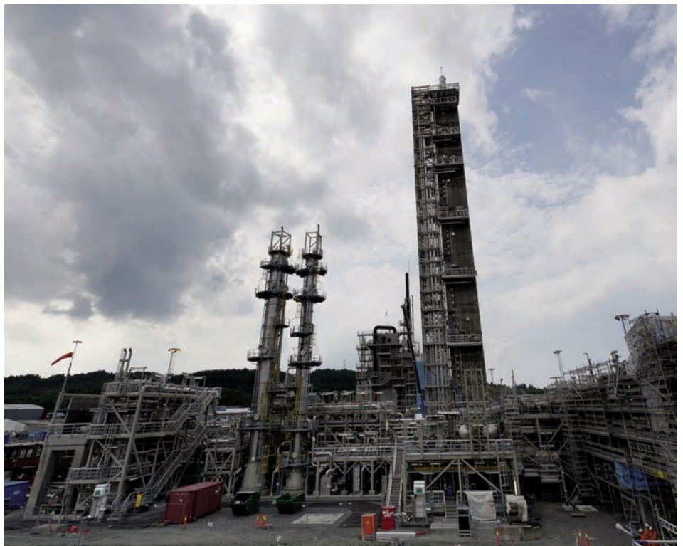
Aker Carbon Capture constructed the TCM absorber present at the technology center today. Photo: Styrk Fjærtøft
