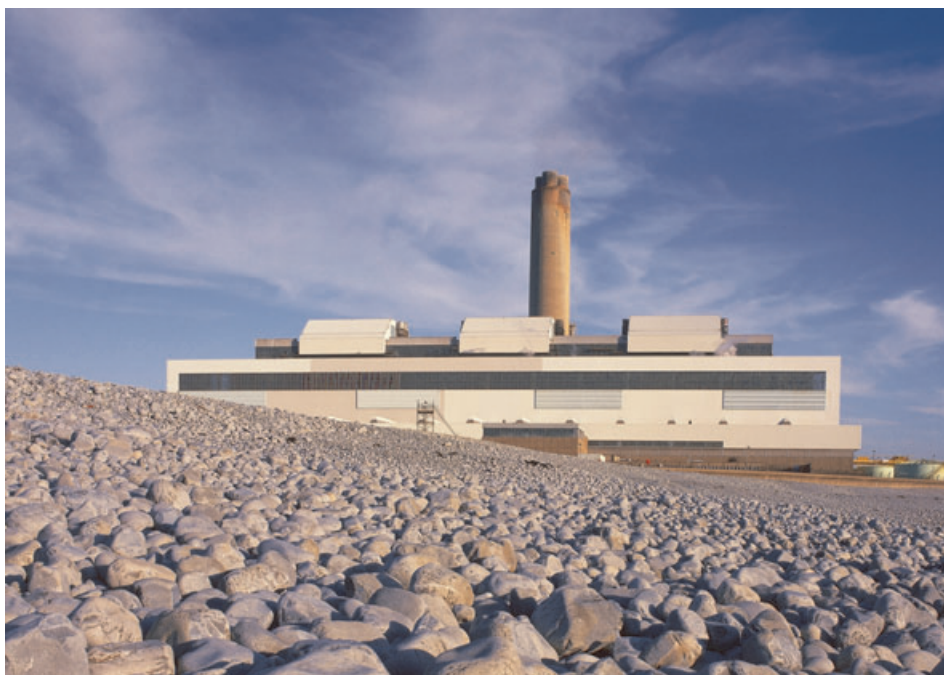
Aberthaw Power Station in Wales, site of the RWE nPower carbon capture pilot that began capturing CO 2 in January
