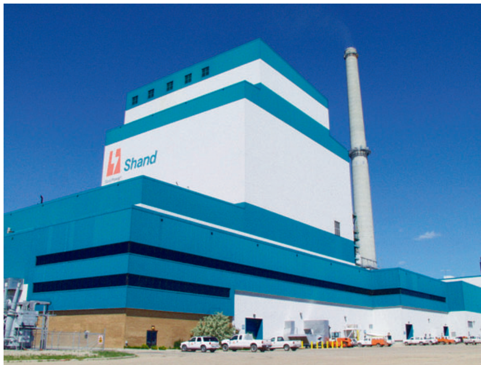
SaskPower's Shand power station will host Hitachi's Carbon Capture Test Facility (©SaskPower)
