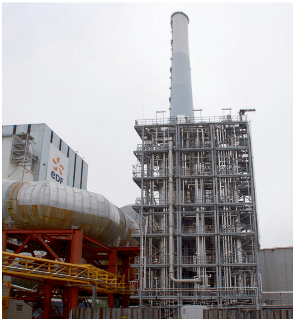
The EDF power plant in Le Havre, France is testing Alstom's carbon capture technology
