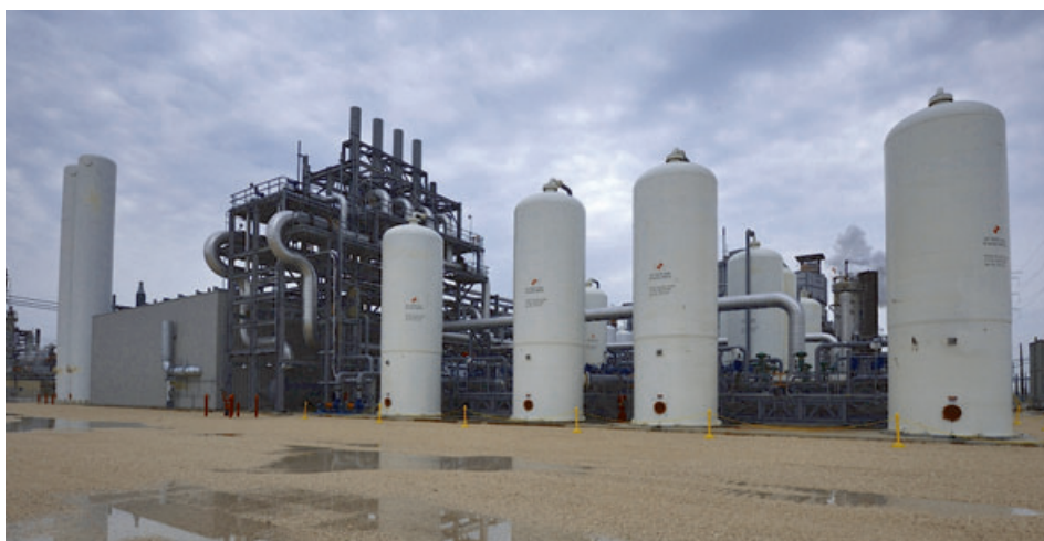
Air Products' Port Arthur CO 2 capture facility in Texas has begun capturing CO 2 (Image courtesy of Air Products and Chemicals, Inc.)
