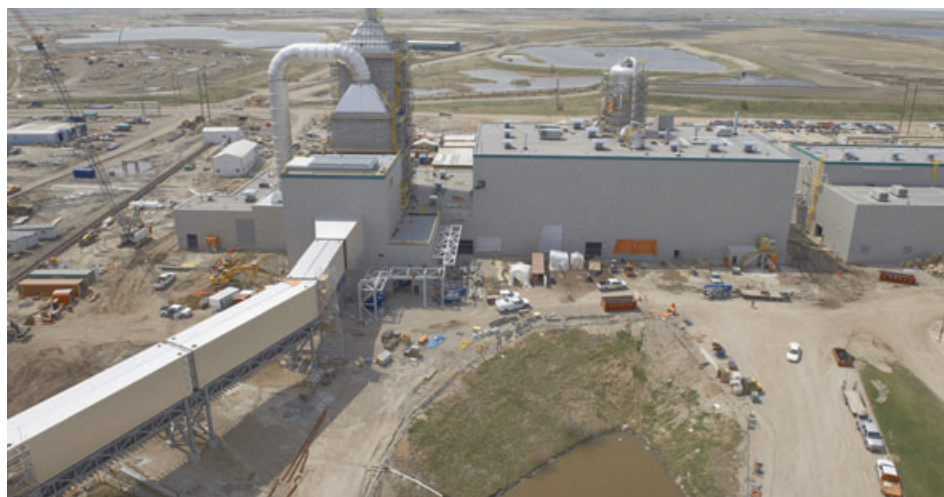
SaskPower's Boundary Dam project is on schedule despite delays and cost overruns - the image shows flue gas ducting running to the carbon capture plant (©Mark Greschner)
