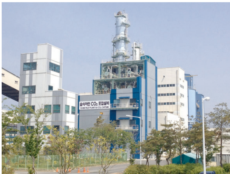
Figure 2 - the 10 MW scale post-combustion CO 2 capture plant
