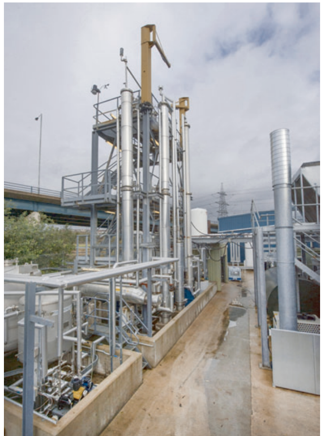
Figure 4a - The PACT core facilities at Beighton include a CO 2 amine capture plant which can treat real flue gas produced by an air combustion/oxyfuel plant or carefully specified gas mixtures produced by on-site gas mixing facilities
