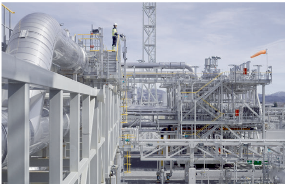
The first phase of testing at Technology Center Mongstad, with technology from Aker and Alstom, is complete and Shell Cansolv has just signed up to test its Carbon Capture System in a new phase
