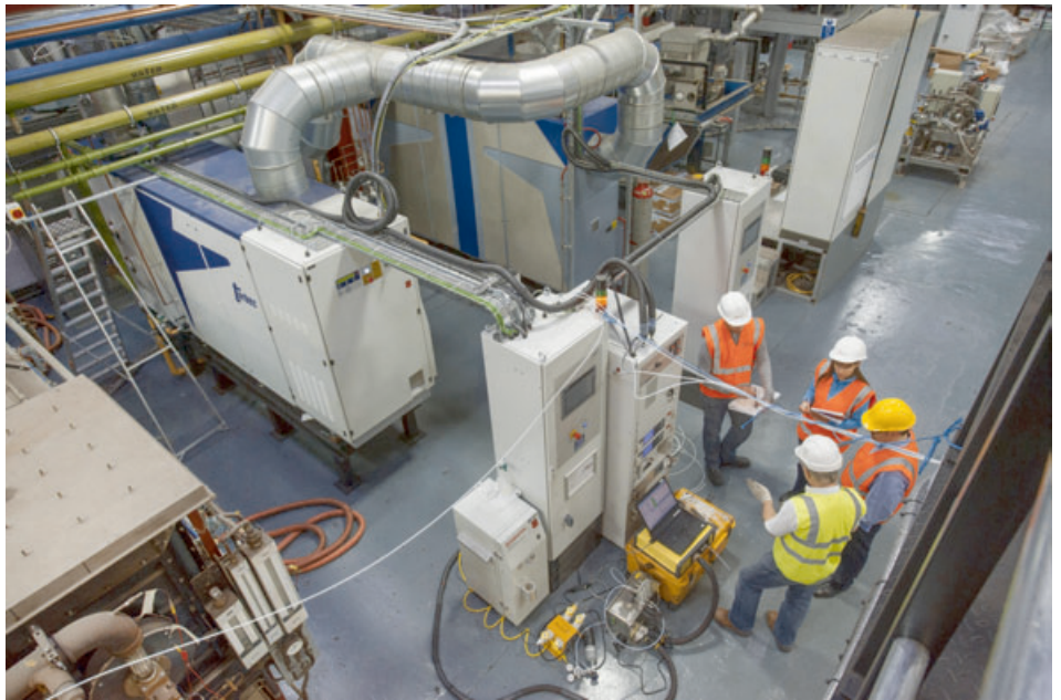
Quantitech's FTIR gas analyser is being used at the UK's Pilot-scale Advanced Capture Technology (PACT) facility
