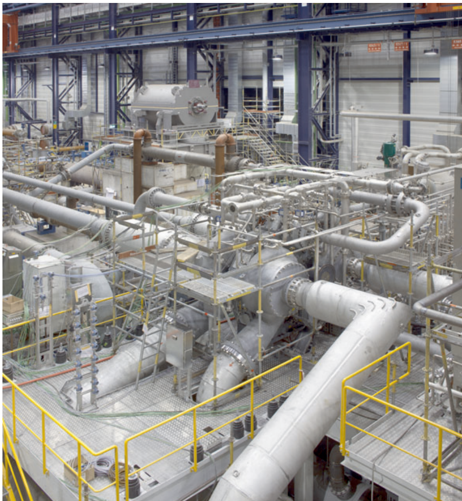
The Siemens compressor at Mississippi Power's Kemper County IGCC project operates at 150 bar and flow of 63,000 m 3 /h
