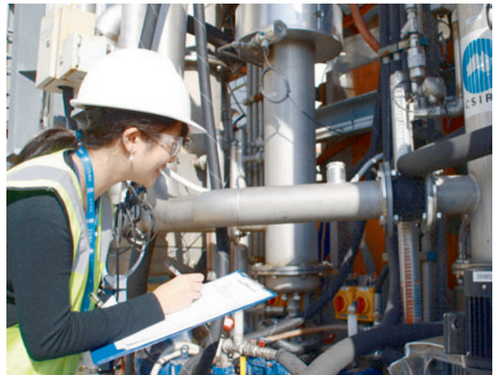
Monash University PhD-student, Mai Bui, records data from CSIRO's existing post-combustion carbon capture pilot plant located at the AGL Loy Yang brown coal power station in the Latrobe Valley, Victoria; image courtesy of CSIRO
