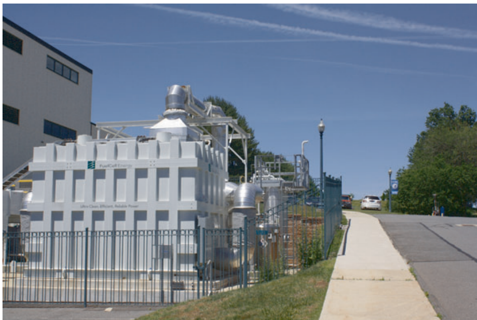
A FuelCell Energy installation – the company's Direct FuelCell technology can be used to capture power plant emissions while also producing additional power
