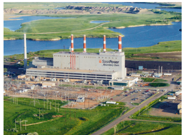
SaskPower's Boundary Dam power station
