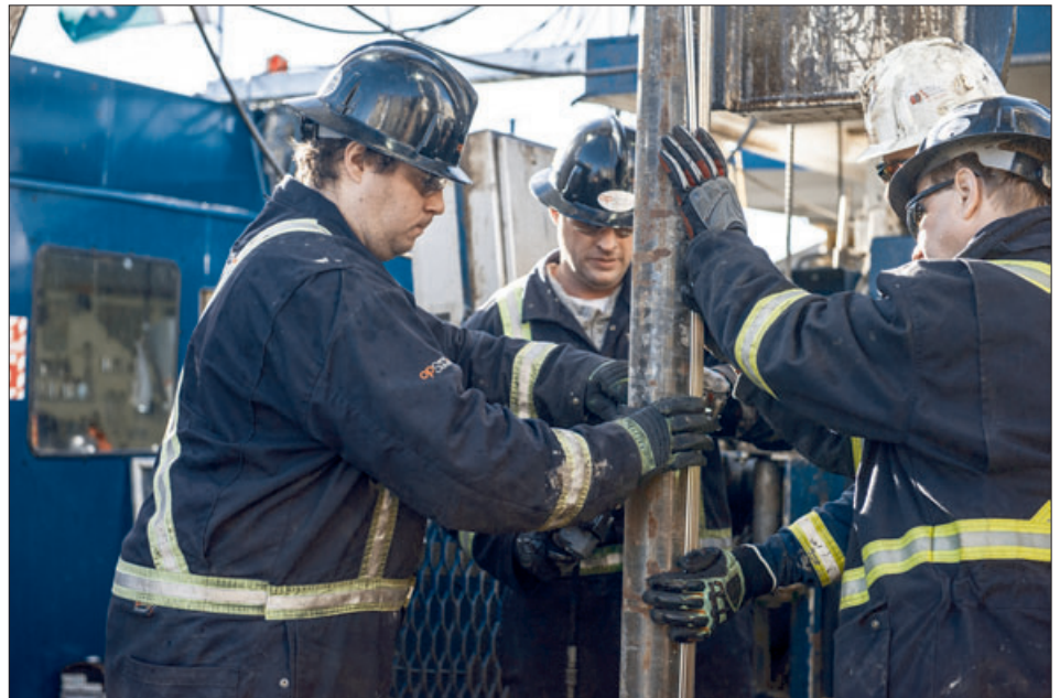
Casing conveyed equipment being installed during the drilling of the Aquistore well
