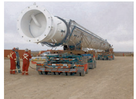
Column transportation to the site
