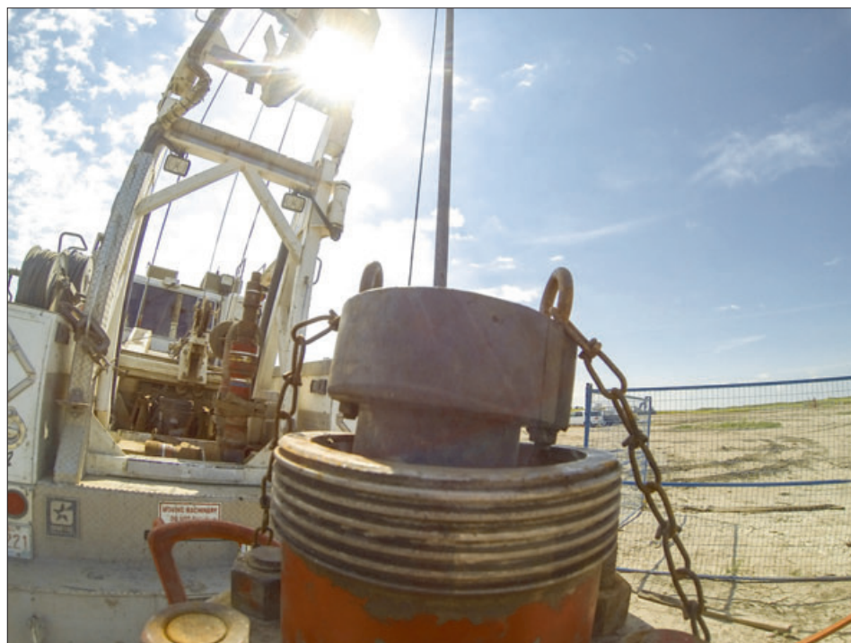
Well logging at the Aquistore project
