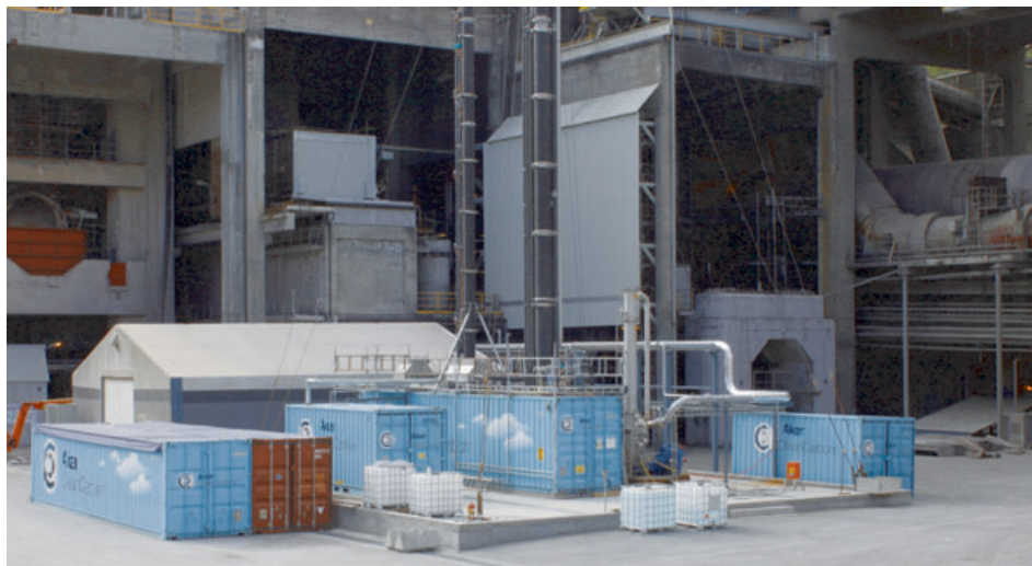
Aker Solutions' Mobile Test Unit (MTU) which was operated for eighteen months in a test campaign at Norcem
