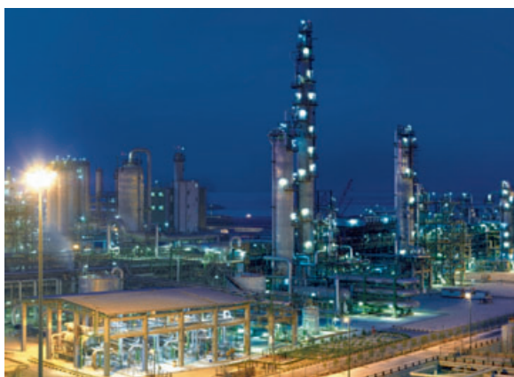
150000 tonnes per day of CO2 will be recovered and reused from an Ethylene Oxide plant in southern Iran
