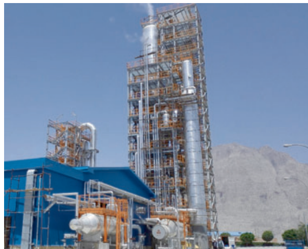
Kermanshab Urea Plant: CO2 is recovered from a gas turbine stack and used to supply a feed stock to manufacture urea, the plant was designed and installed by an Iranian manufacturer
