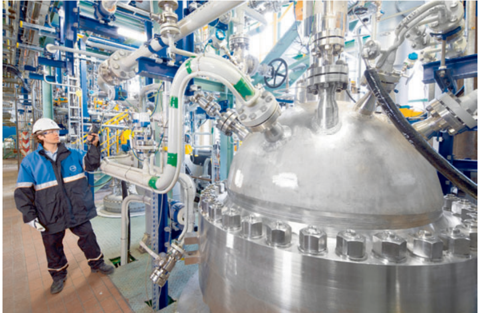
Carbon dioxide as new raw material: At this production plant in Dormagen, Covestro is now incorporating 20 percent CO 2 into an important foam component (Image ©Covestro)
