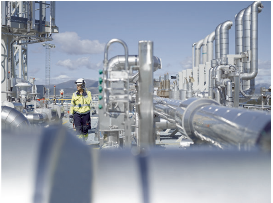
ION Engineering is testing its solvent at Technology Centre Mongstad as the next step towards commercialisation
