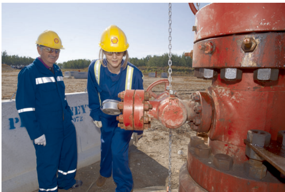
CO 2 injection at the Quest site. Shell has developed a detailed measurement, monitoring and verification plan that includes atmospheric, biosphere, hydrosphere, geosphere and well-based monitoring at its Quest project (Image ©Shell)
