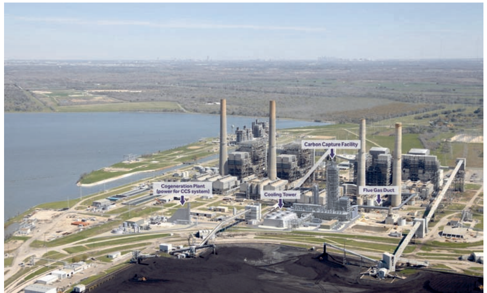
Petra Nova applies carbon capture technology to an existing unit at the coal-fired W.A. Parish Generating Station (Image: ©NRG Energy)
