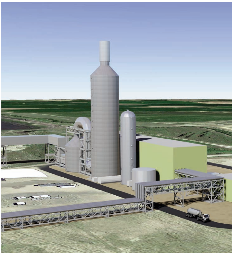
Figure 1 - The conceptual 300 MW CO 2 capture island and supporting balance of plant systems
