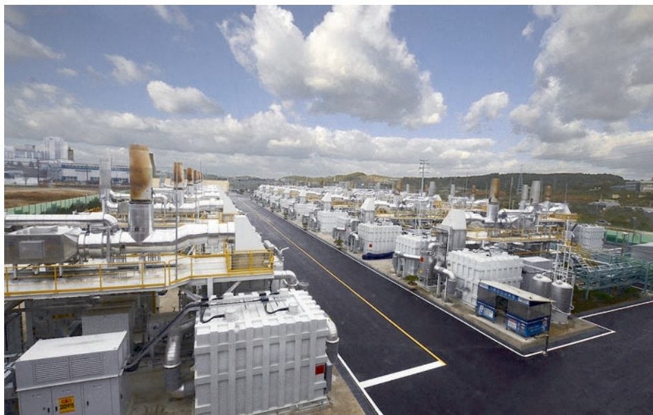
FuelCell Energy's largest carbon fuel cell plant, based near Seoul, uses 21 four stack modules, generating 1.4 MW
