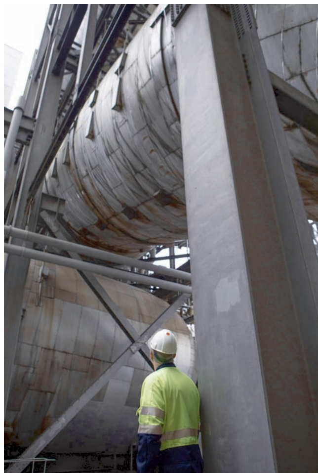
An engineer looks up at flue gas desulphurisation unit (FGD) at Drax Power Station. The massive pipe would transport flue gas from the Drax boilers to the carbon capture and storage (CCS) plant for CO 2 removal of between 90-95%
