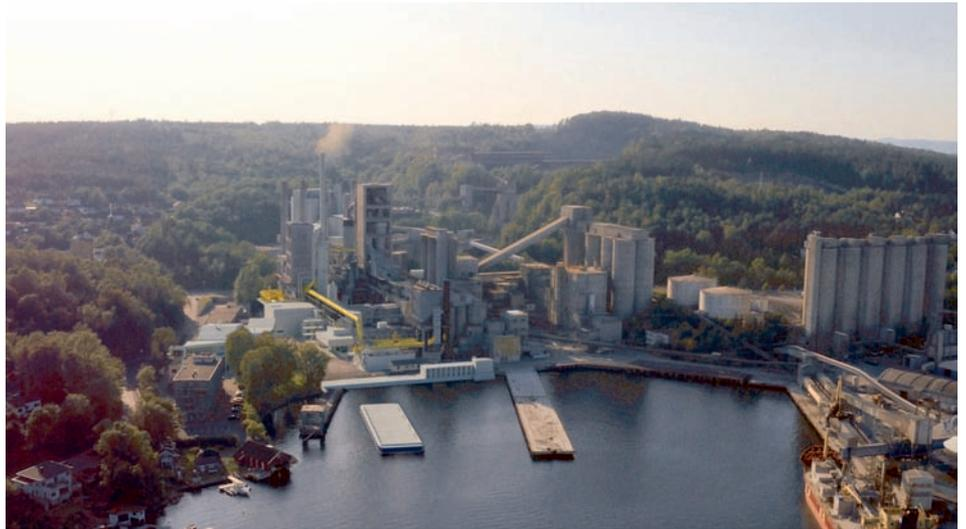
*The Brevik CCS project will enable the capture of 400,000 tonnes of CO<sub>2</sub> per year and the transportation for permanent storage, making it the first industrial-scale CCS project at a cement production plant in the world*
