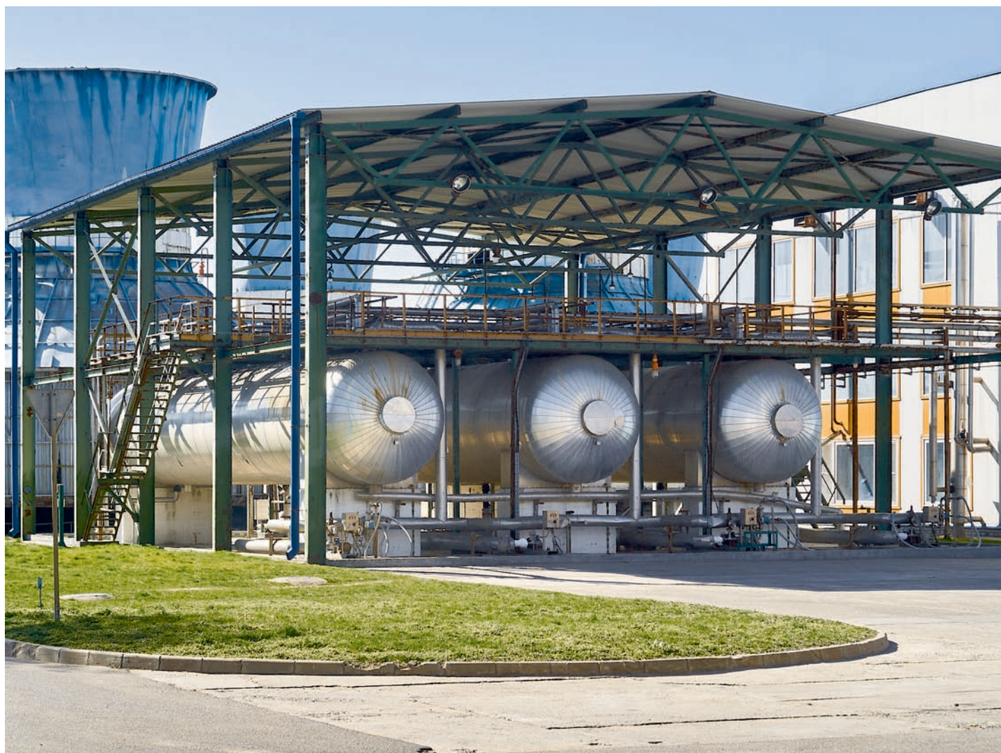
Cryogenic liquid CO 2 storage tanks
