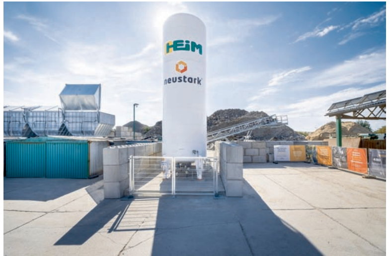
Neustark's CO 2 storage site in Berlin has the capacity to store 1,000 tons of CO 2 per year captured from biogas plants
