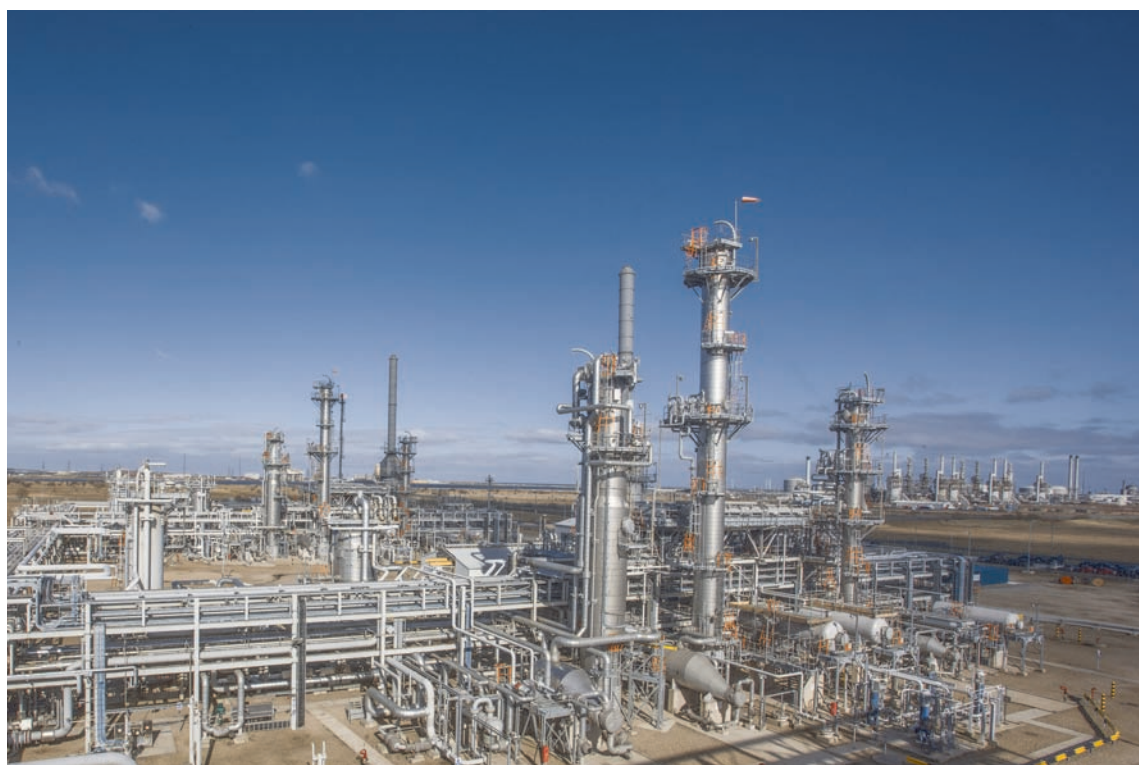
Kellas' CATS (Central Area Transmission System) gas processing terminal in Teesside will deliver 355MW of hydrogen in Phase 1 to Statera's Saltholme power stations
