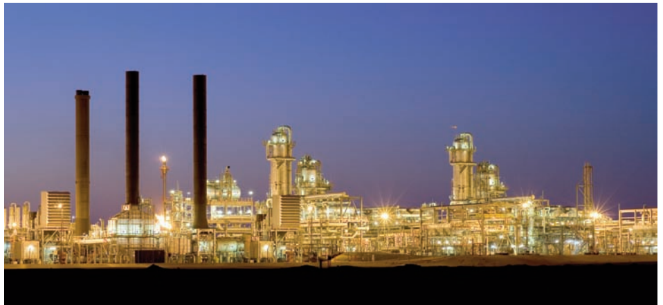
The In Salah CCS project in central Algeria is a world pioneering onshore CO 2 capture and storage project which has built up a wealth of experience highly relevant to CCS projects worldwide. Carbon dioxide from several gas fields is removed from the gas production stream in a central gas processing facility and then the CO 2 is compressed, transported and stored underground in the 1.9 km deep Carboniferous sandstone unit at the Krechba field
