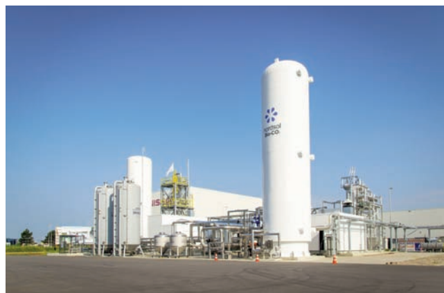
Nordsol opened the first Dutch bio-LNG plant in October 2021 with Renewi and Shell. This plant upgrades and liquefies 8 million Nm 3 biogas from organic waste into 3.4 kilotons of bio-LNG and 6.3 kilotons of biogenic liquid CO 2 per year
